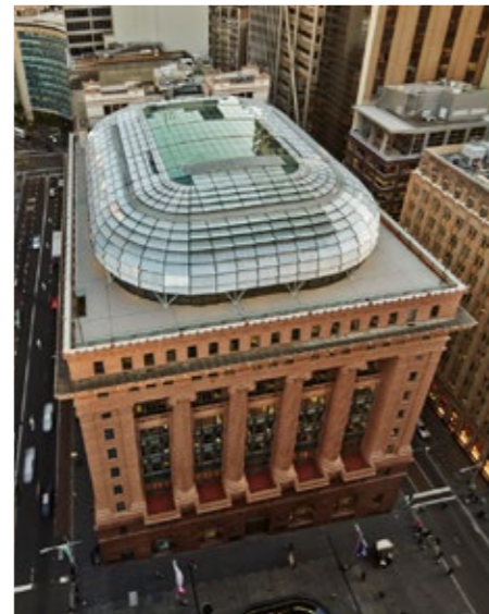
50 Martin Place \ This iconic building showcases innovation and creativity in engineering solutions, and is considered a masterpiece of sustainable innovation with its maximum Green Star rating
