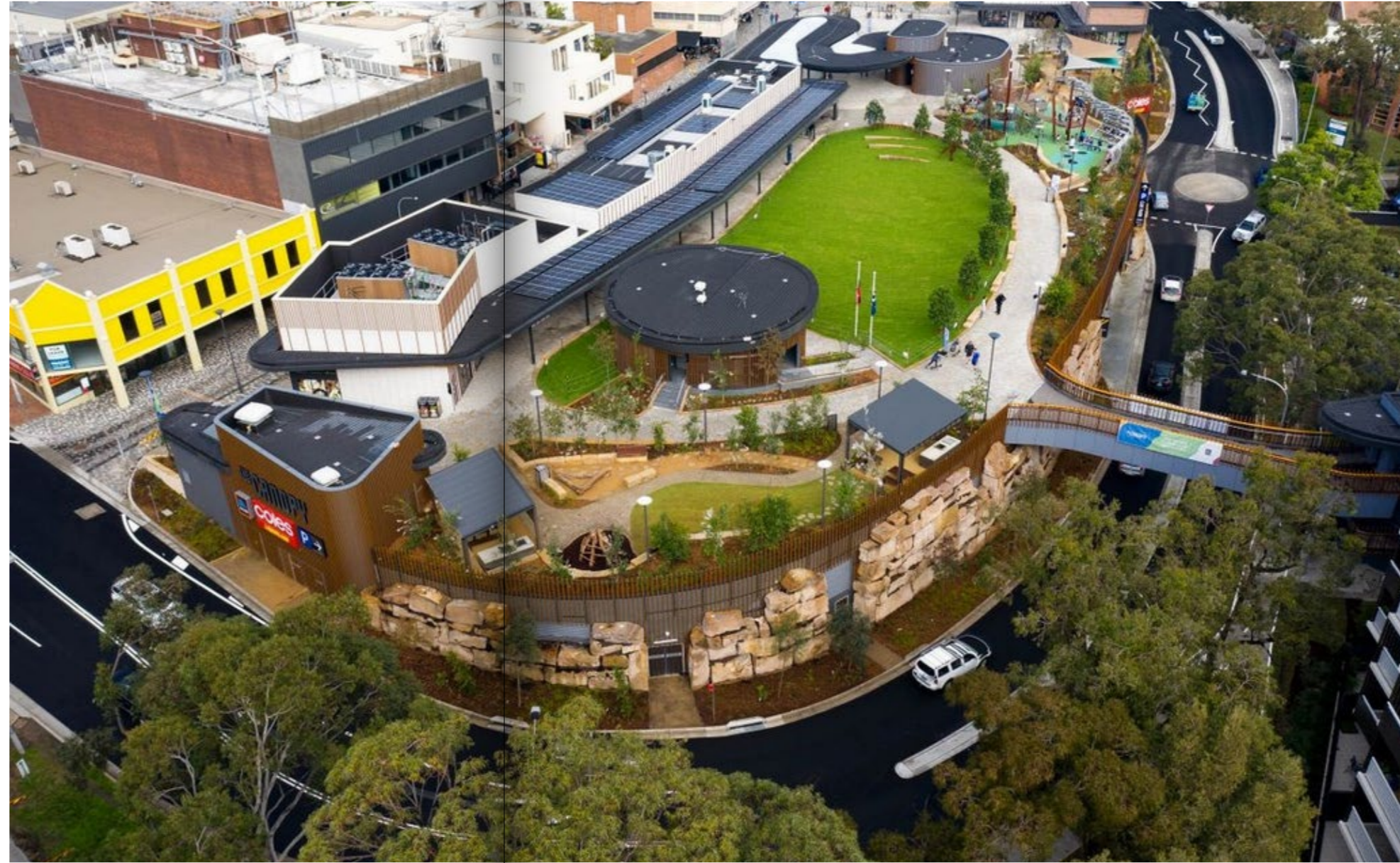
The Canopy, Lane Cove \ TTW provided structural, civil and traffic services for the Canopy in Lane Cove, NSW. This project replaced an existing car park with a new village green, playground, restaurant precinct.
